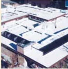
Conklin's Fabric-Reinforced roofing system is extremely versatile and can be applied to many different types of roofs. A Conklin contractor will cover the proper procedure for application of our Fabric-Reinforced system to your particular roof substrate.
